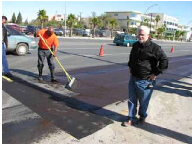
Rubberized Emulsion Aggregate Slurry (REAS) was applied to miles of hurricane-ravaged pavement in Juarez, Mexico.
